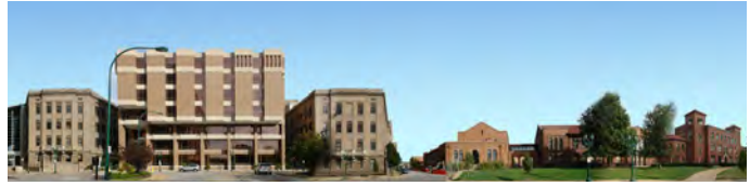
Euclid Avenue - West Facades
