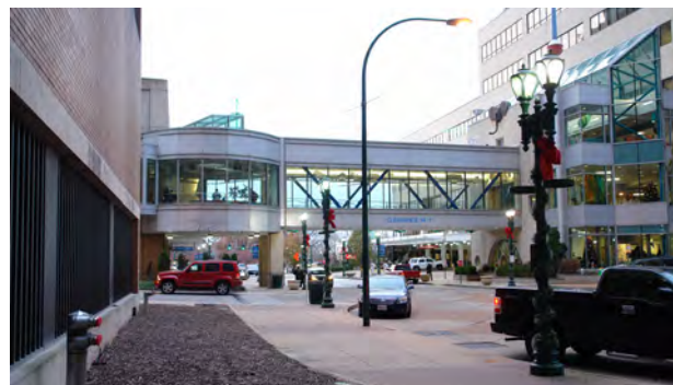
Link over Children's Place at Building #49 - West Face
