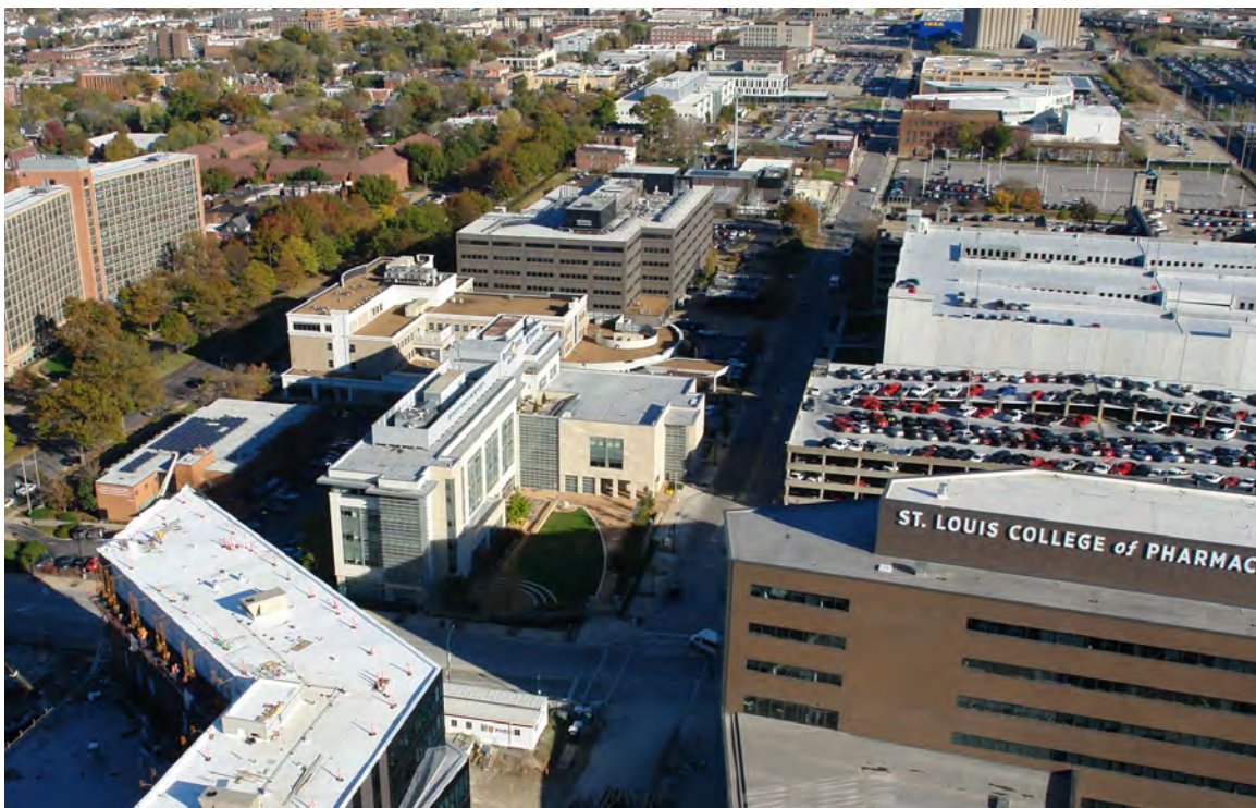
West Aerial View of Tier 3. The Goldfarb School of Nursing is seen with the 4444 Building in the background.
