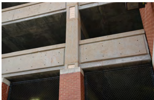
Pre-Cast Concrete, Brick
