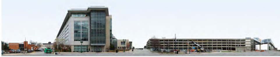
Taylor Avenue - West Facades
