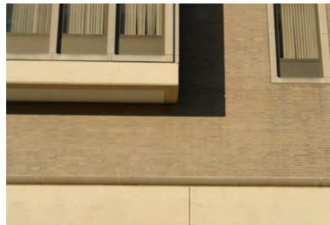
Brick, Limestone, Pre-Cast Concrete, Glazing
