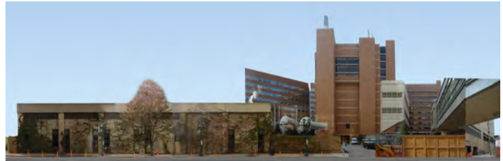
Parkview Place - North Facades
