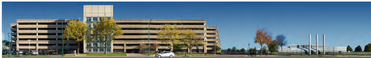
Clayton Avenue - South Facades
