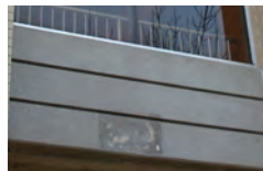
Exposed Aggregate Pre-Cast Concrete
