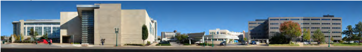
Duncan Avenue - South Facades
