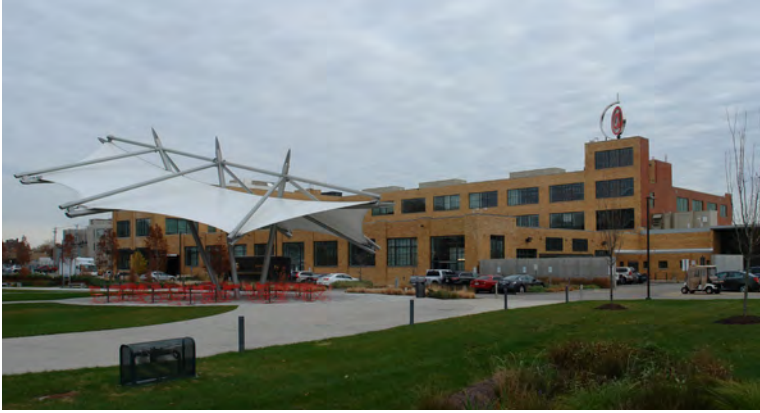
Building 537 @4240, Southwest Facade
