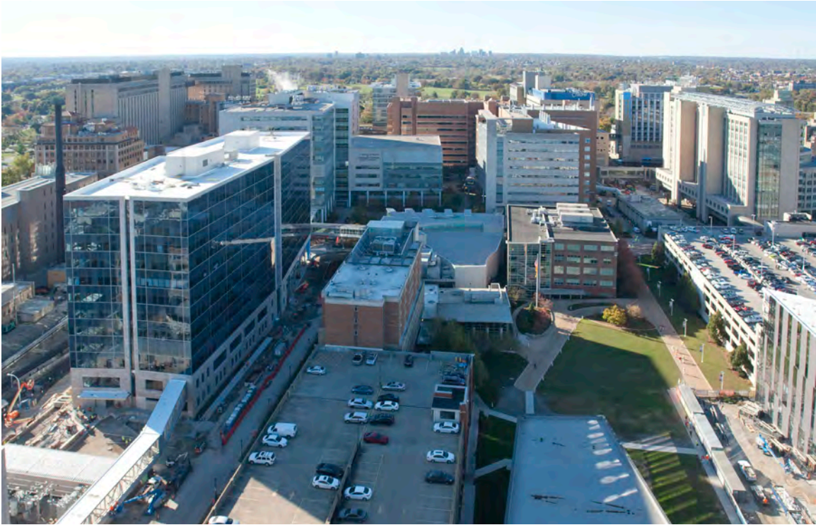
East Aerial View of Tier 1. The new MCC in Tier 2 is seen in the foreground with Hope Plaza bounded by the MPRB and BJCIH. CSRB is beyond.
