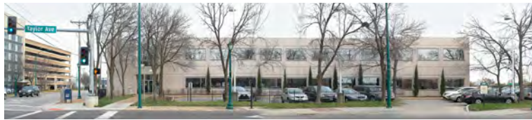
Taylor Avenue - West Facades
