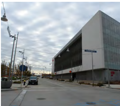
Boyle Ave. - View South
