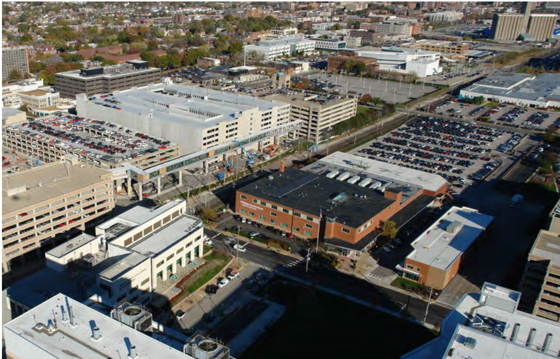
Northwest Aerial View of Tier 3. The Institute for Public Health and surrounding structured and surface parking.
