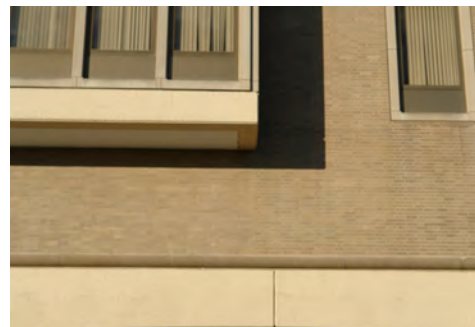
Brick, Limestone, Pre-Cast Concrete, Glazing
