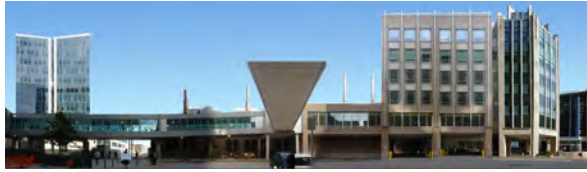
Euclid Avenue - West Facades
