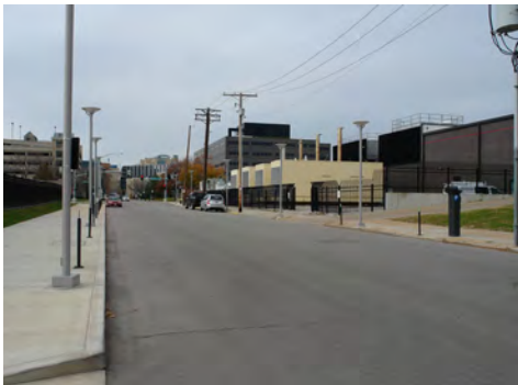
Duncan Ave. - View West
