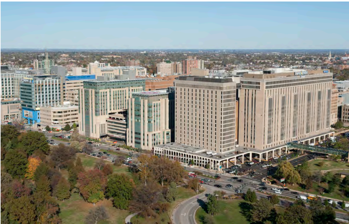
Southwest Aerial View of Tier 1. Details within the tan and buff palette include bronze and green-blue glazing.
