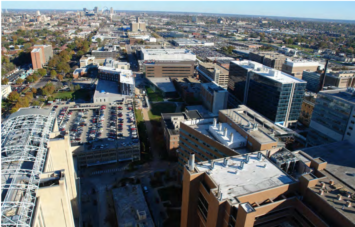
West Aerial View of Tier 2 UHSP campus with MMC to the right, bounding Hope Plaza.
