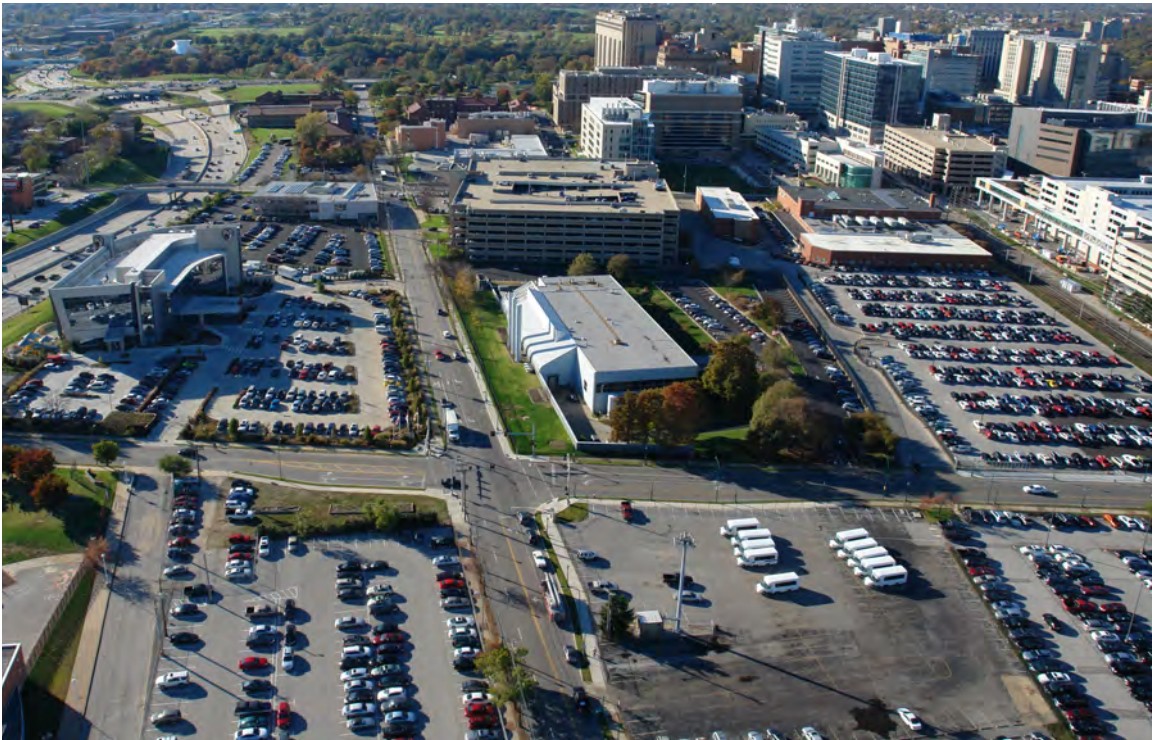
East Aerial View of Tier 3. Shriners' Hospital and the Newstead Facility occupy the southeast portion of Tier 3.
