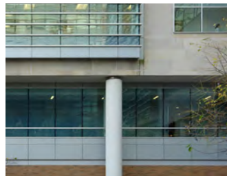
Brick, Limestone, Concrete, Metal, Glazing
