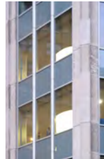
Glazing, Spandrel, Limestone
