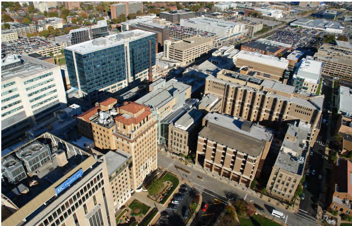
West Aerial View of Tier 2. The tan and brown brick of the School of Medicine are seen on the North and South Buildings as well as Becker Medical Library and McDonnell Sciences.
