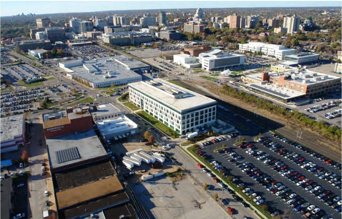
Southwest Aerial View of Tier 4. The BJC Commons can be seen with its surface parking and the Clayton Avenue Building in the background.
