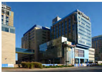
Parkview Place - North Facades
