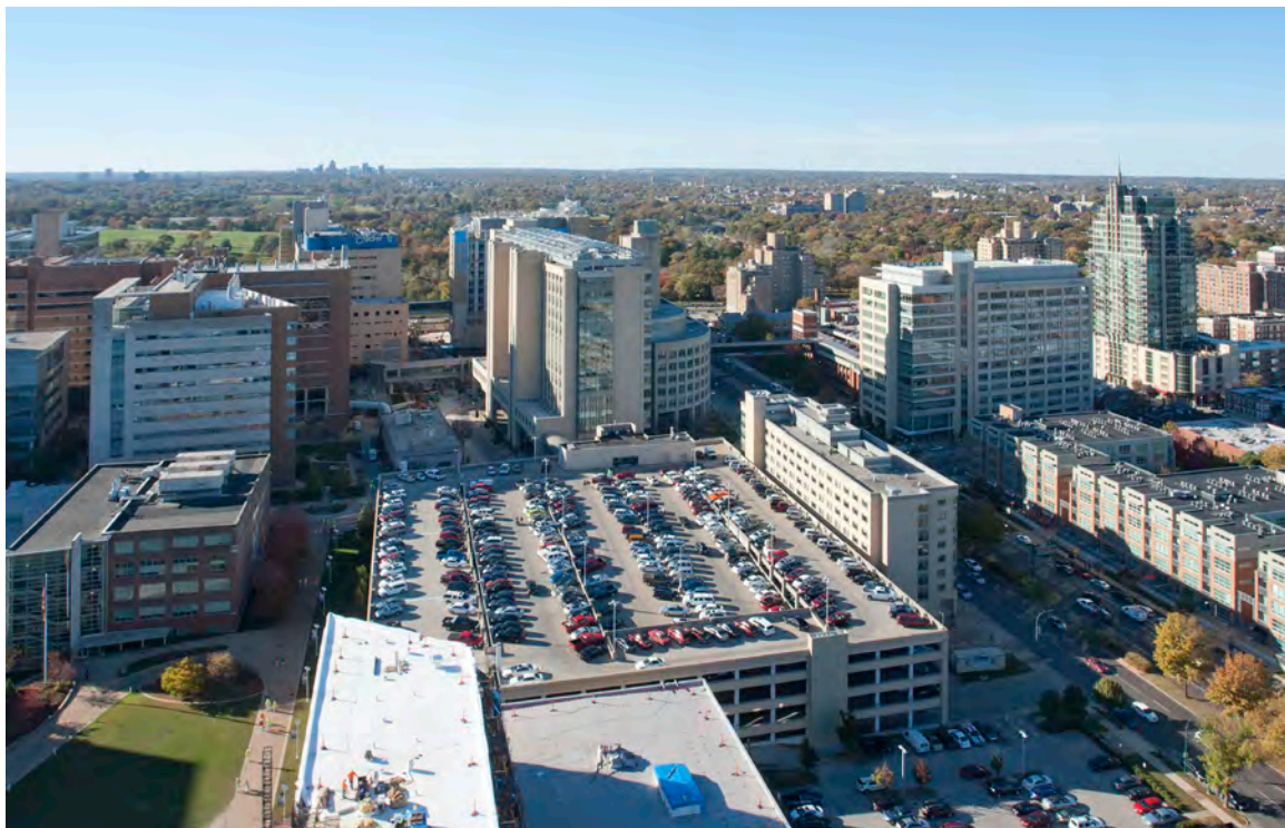
East Aerial View of Tier 1. MPRB, CAM, and COH are seen along the east boundary of Tier 1.
