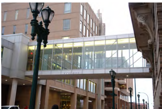
Link over Euclid Ave. at Building #9 - North Face
