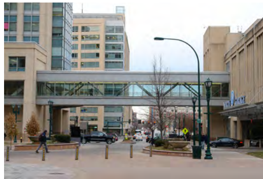
Link over Euclid Ave. at Building #35 - South Face
