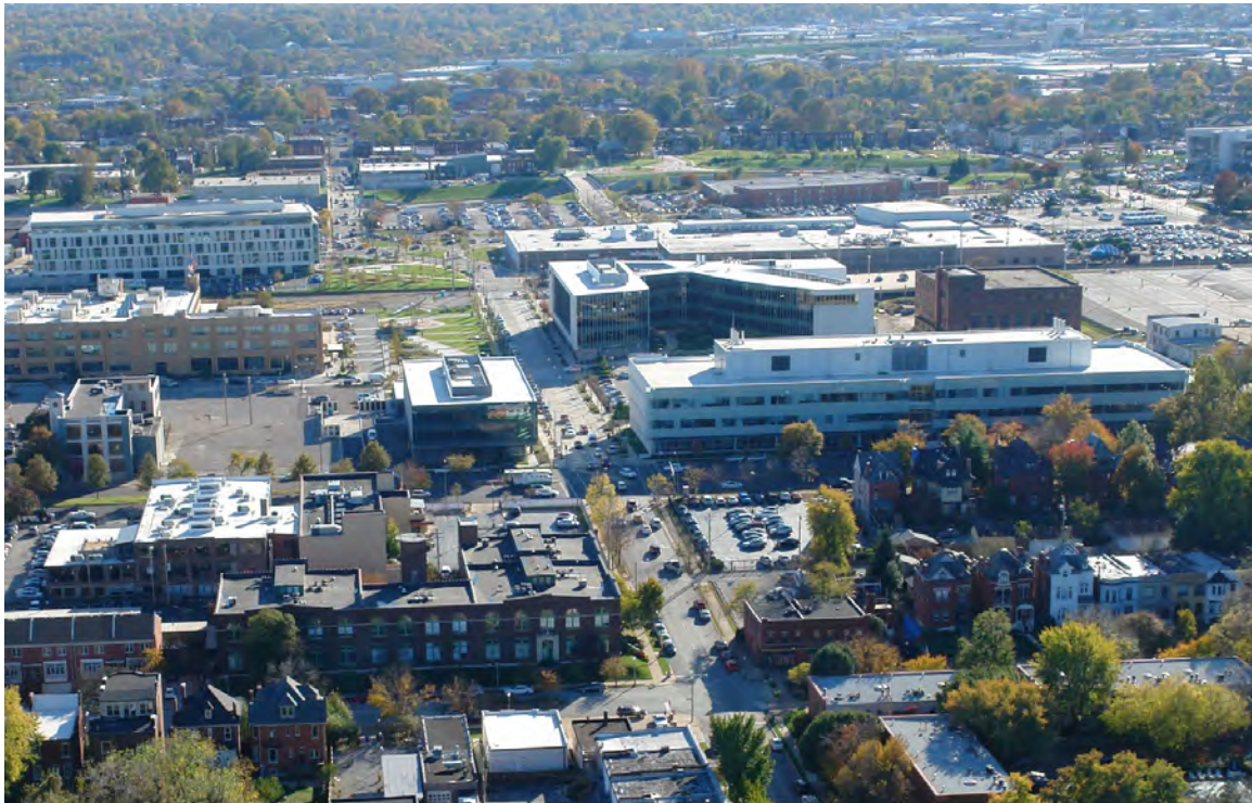
North Aerial View of Tier 4
