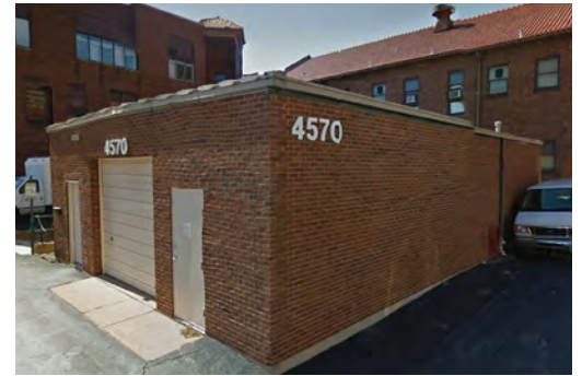
Northeast Facade, Brick
