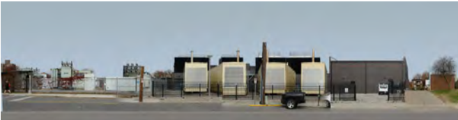
Duncan Avenue - South Facades
