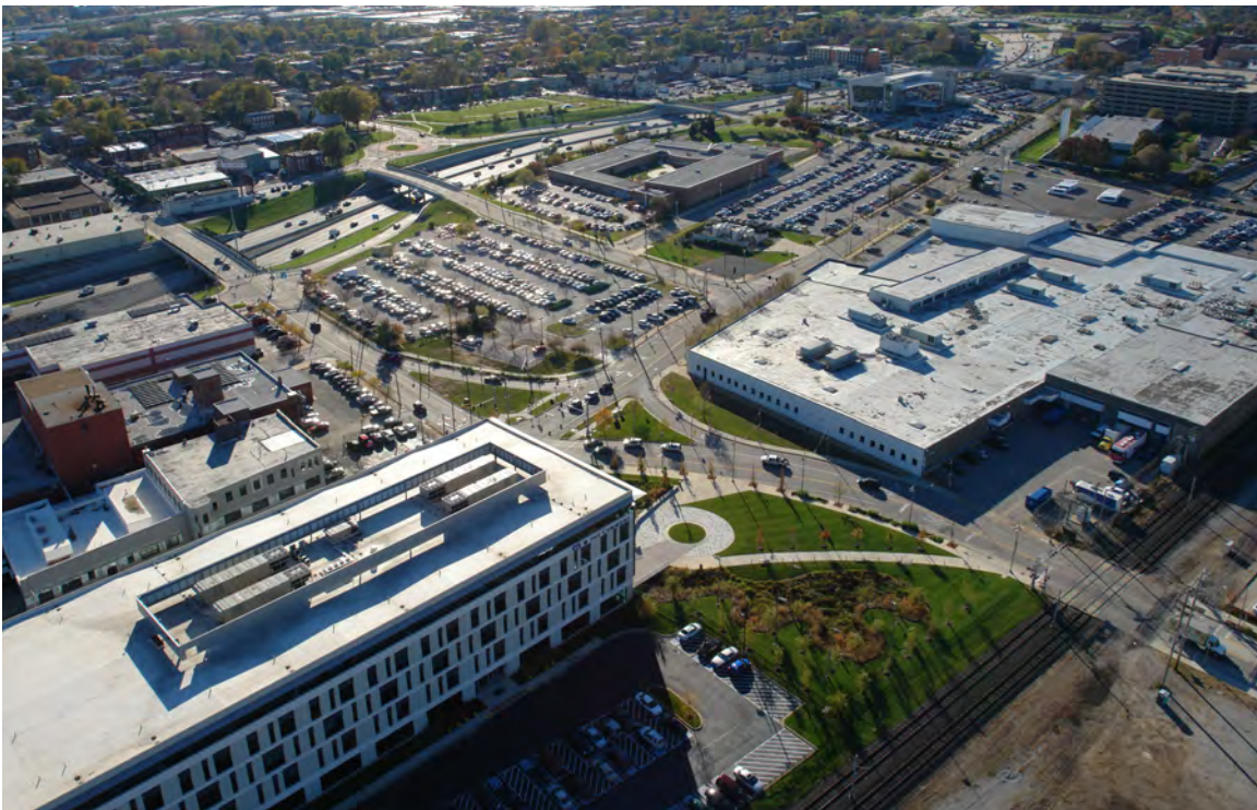
Southwest Aerial View of Tier 4
