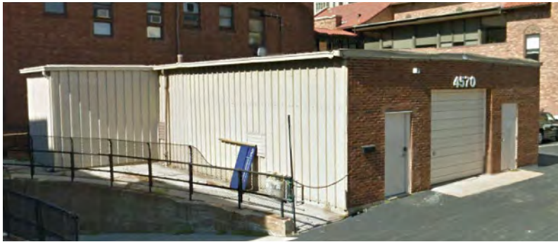
Southeast Facade, Brick, Metal
