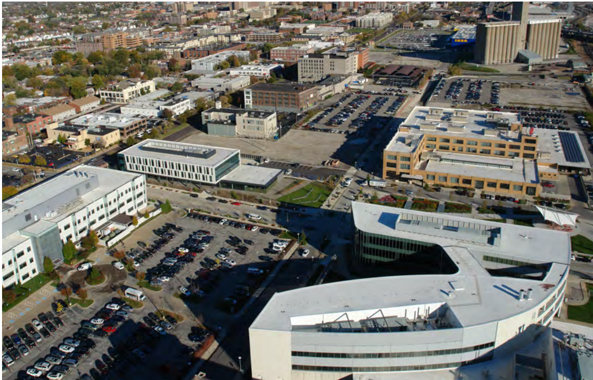
Southwest Aerial View of Tier 4
