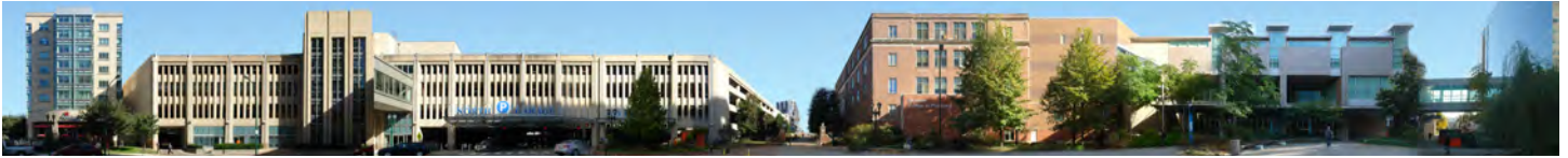
Euclid Avenue - West Facades
