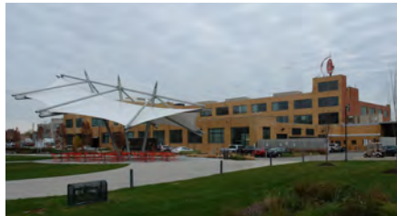
Boyle Avenue - Southwest Facades
