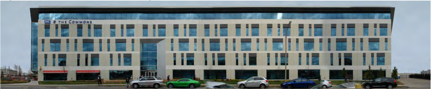
Clayton Avenue - South Facades
