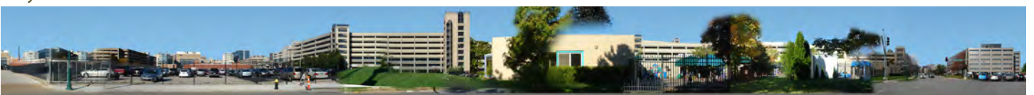
Newstead Avenue - East Facades
