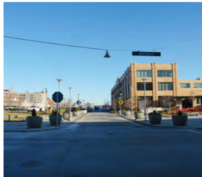
Duncan Ave. - View East
