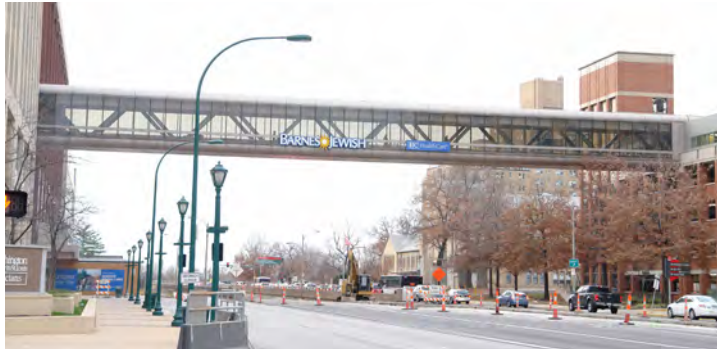
Link over Forest Park Parkway at Building #33 - East Face
