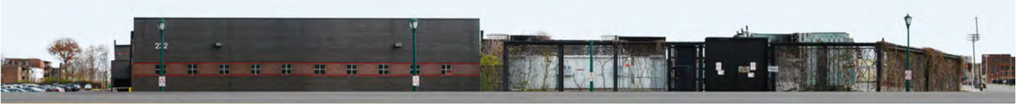
Newstead Avenue - West Facades
