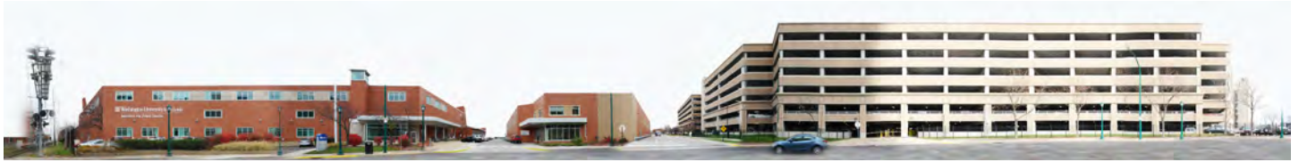
Taylor Avenue - West Facades
