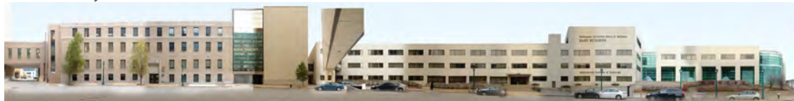
Scott Avenue - South Facades
