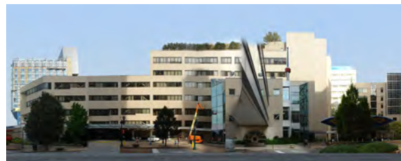
Children's Place - South Facades
