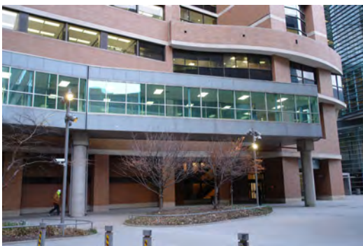
Link at Building #86 - South Face
