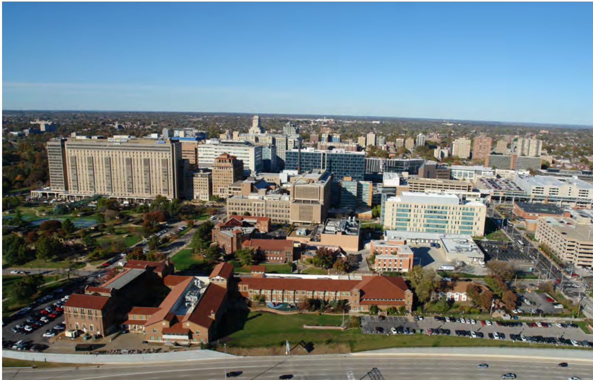
South Aerial View of Tier 2. The CID with its red-orange terra cotta roofs is seen along Hwy. 64/40.
