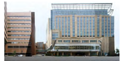
Children's Place - North Facades
