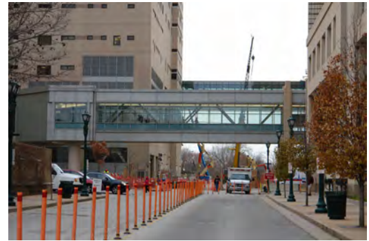
Link over Parkview Place - East Face
